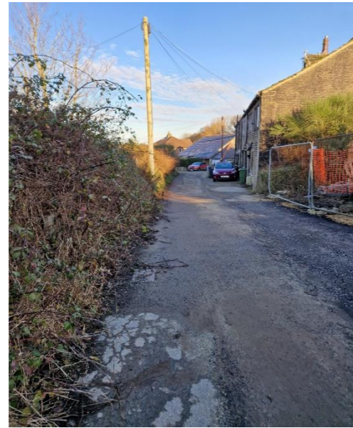
Photo 7: Surface of Application Route fully transitions from earth to tarmac, leading passed residential properties.
